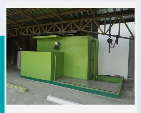
An STP catering to treating domestic wastewater from a textile production line. Located in Valenzuela city, the project requires dealing with low incoming influent wastewater.
